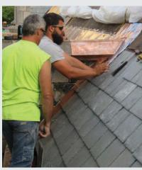
The installation called for a 3-inch head lap. "With random slate, you don't need to put any vertical lines in, because nothing is going to line up vertically," Dennison explains. "Every side lap has to be at least 3 inches, but there is no set pattern for the widths-we just mix them up. That's why they use the term 'random."
