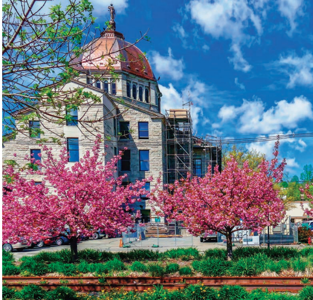
Bradford County Courthouse’s new copper dome
